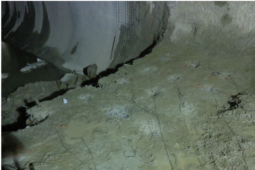
Capsules triggered by electrical currents
