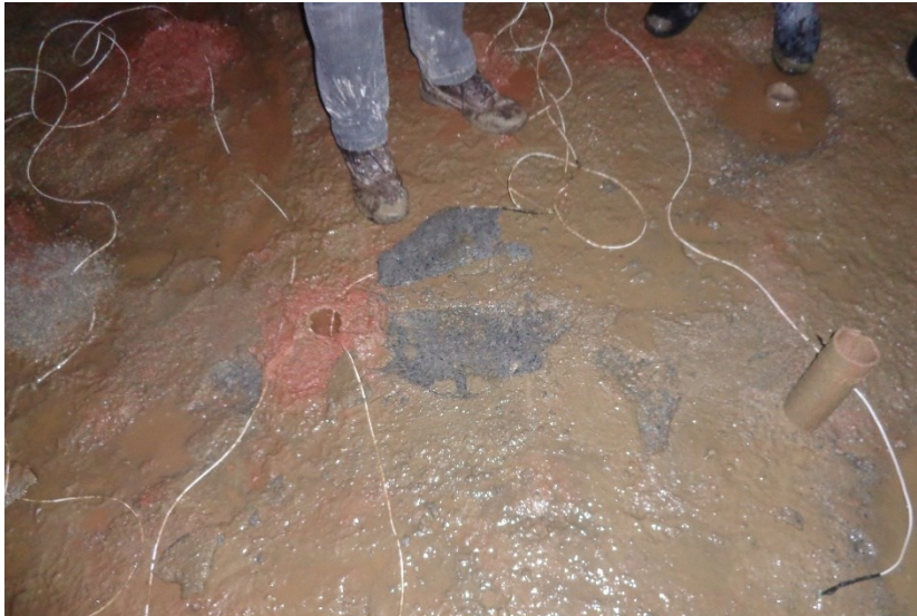
Holes bored in the rock
