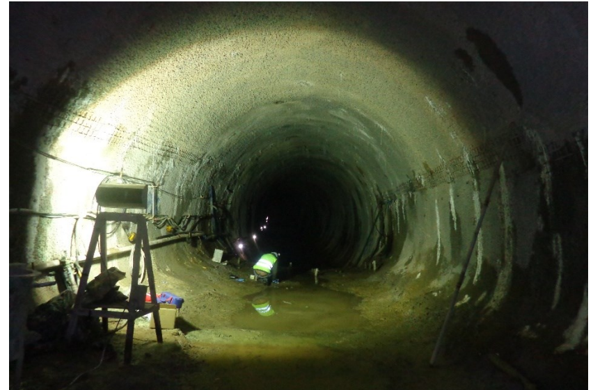
Shallow NATM tunnel
