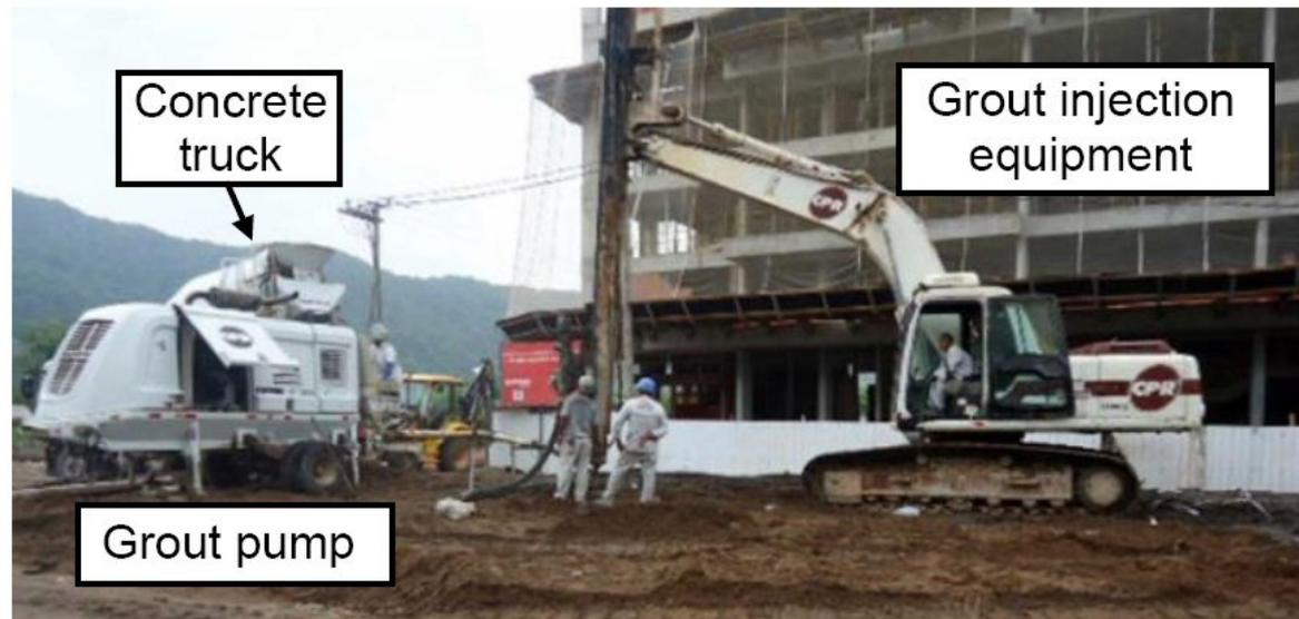
Figure 2. Grouting work in progress at Pontal Oceânico.
