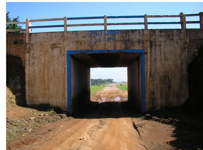
Underpass with a span of less than 5 meters
