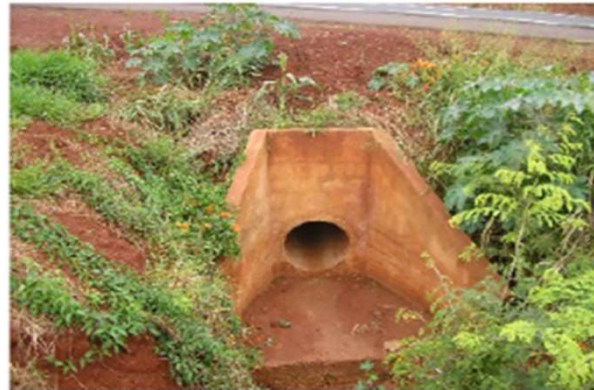
Figure 1. Examples of rainwater gallery inspected (source: IPT)
