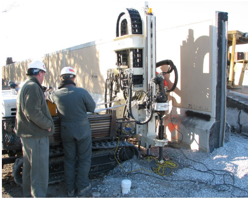
Figure 3: Geoprobe CPT rig at Levee Concrete Wall on Sheet Pile
