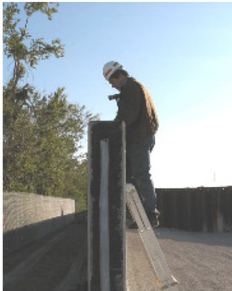
Figure 5: Impacting the Top of the Levee Wall
