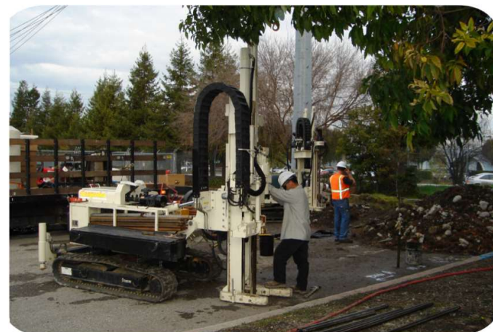
Injection of vegetable oil underground to improve conditions for bioremediation.
