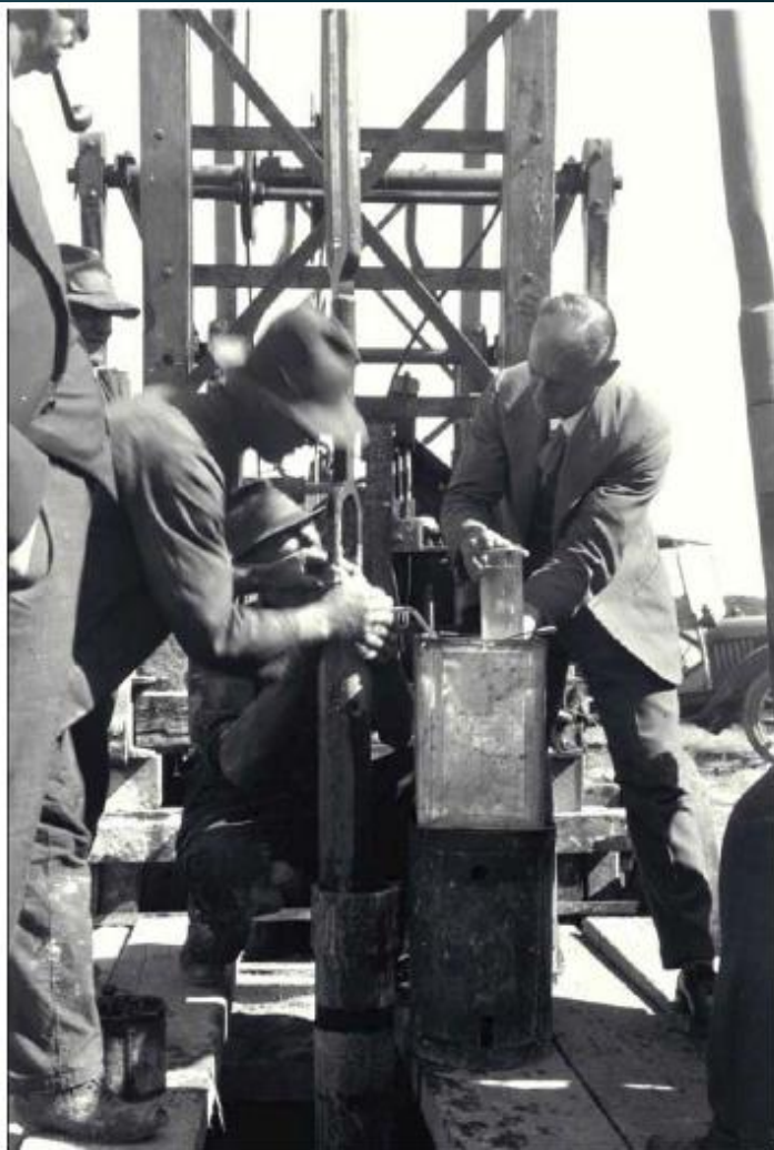
Collecting gas from the Ramsay Oil Bore 1 near Minlaton in 1931. The well reached ~550m, and a small gas flow of almost pure hydrogen was recorded.
